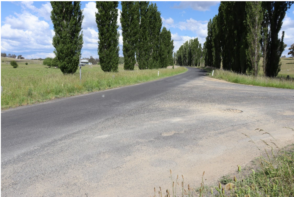
Photograph 27 – Newsomes Road / Wellington Vale Road Intersection (Throat wear left out)
