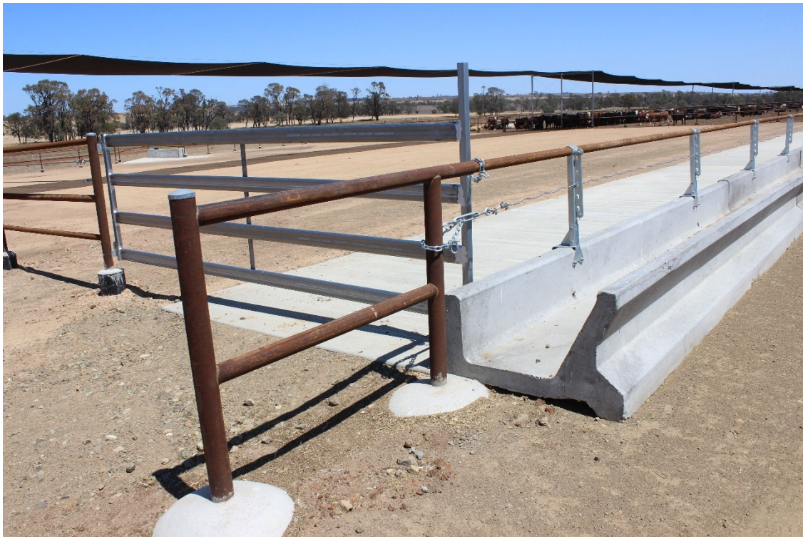
Photograph 12 – Typical pre-cast concrete open feed bunk
