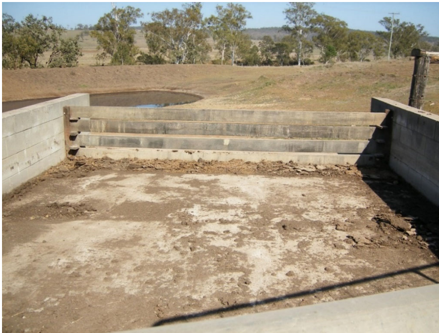
Photograph 13 – Sedimentation basin control outlet – Horizontal drop-board weir
