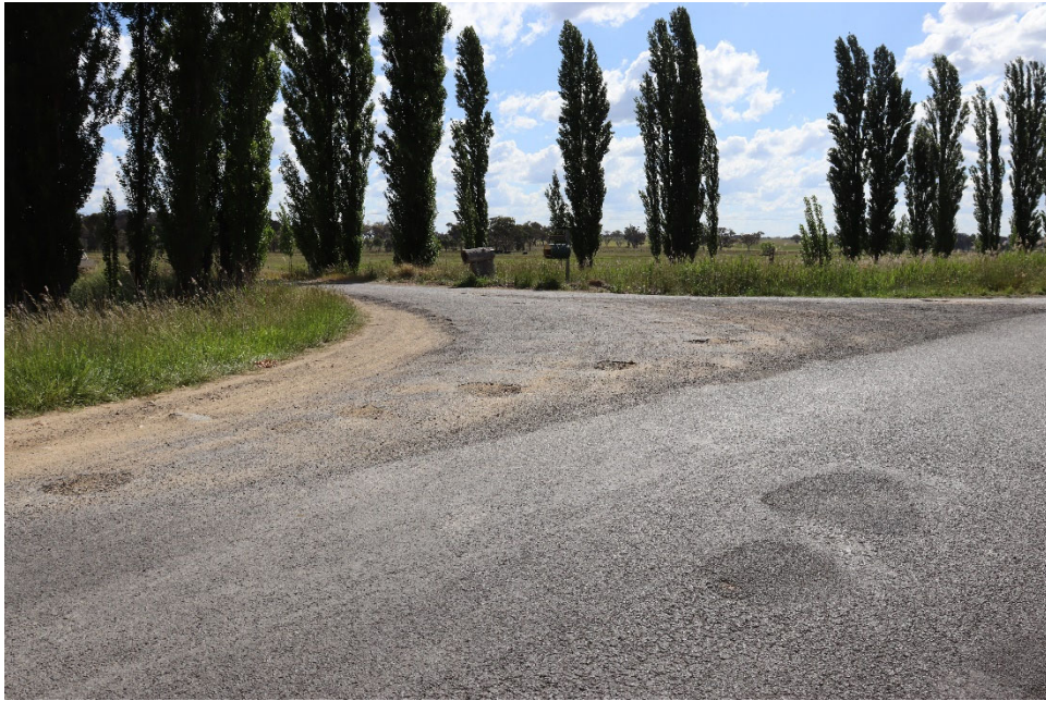
Photograph 26 – Newsomes Road / Wellington Vale Road Intersection (Throat wear right out)
